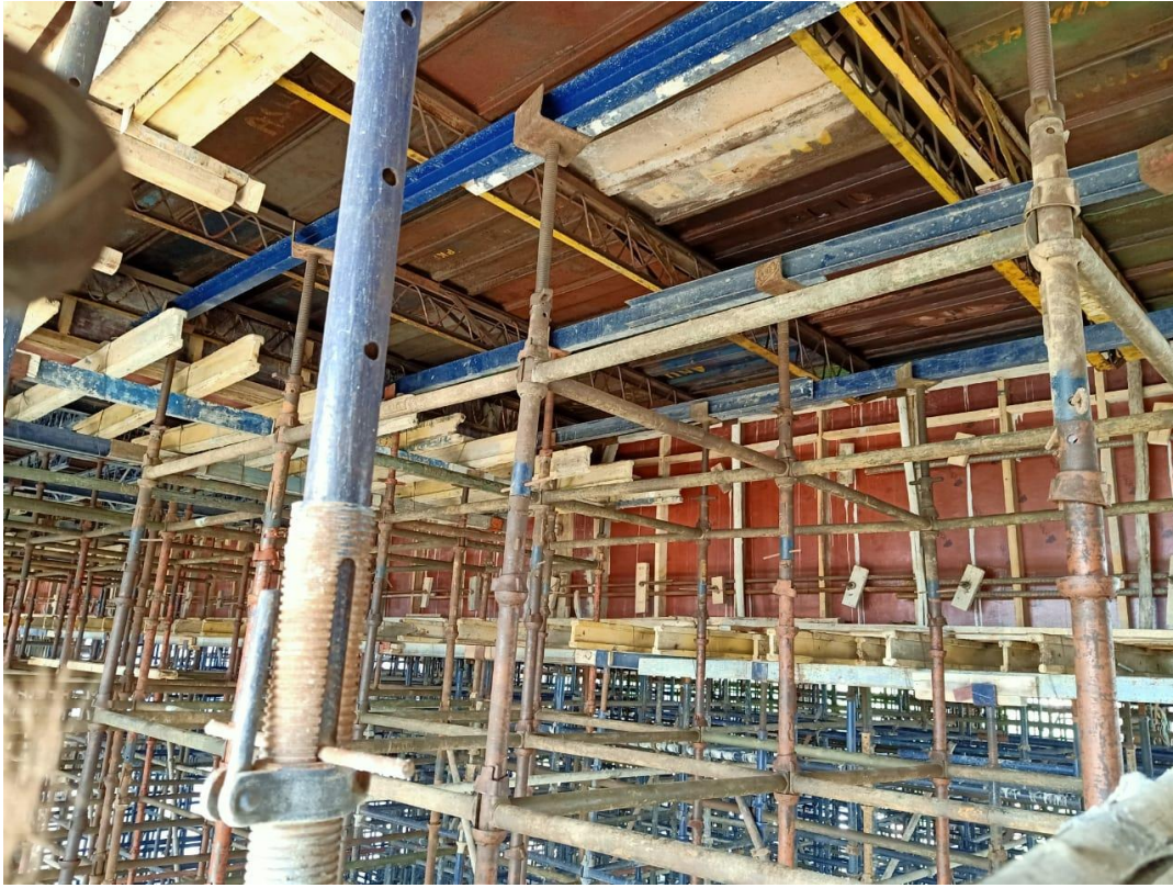
Shuttering work for post tensioning beam
