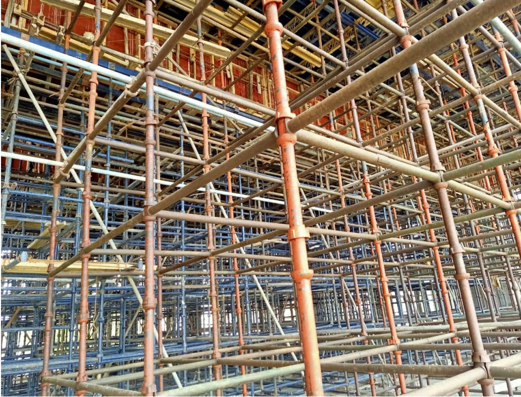
Shuttering work for Pre stressing Beam and Slab
